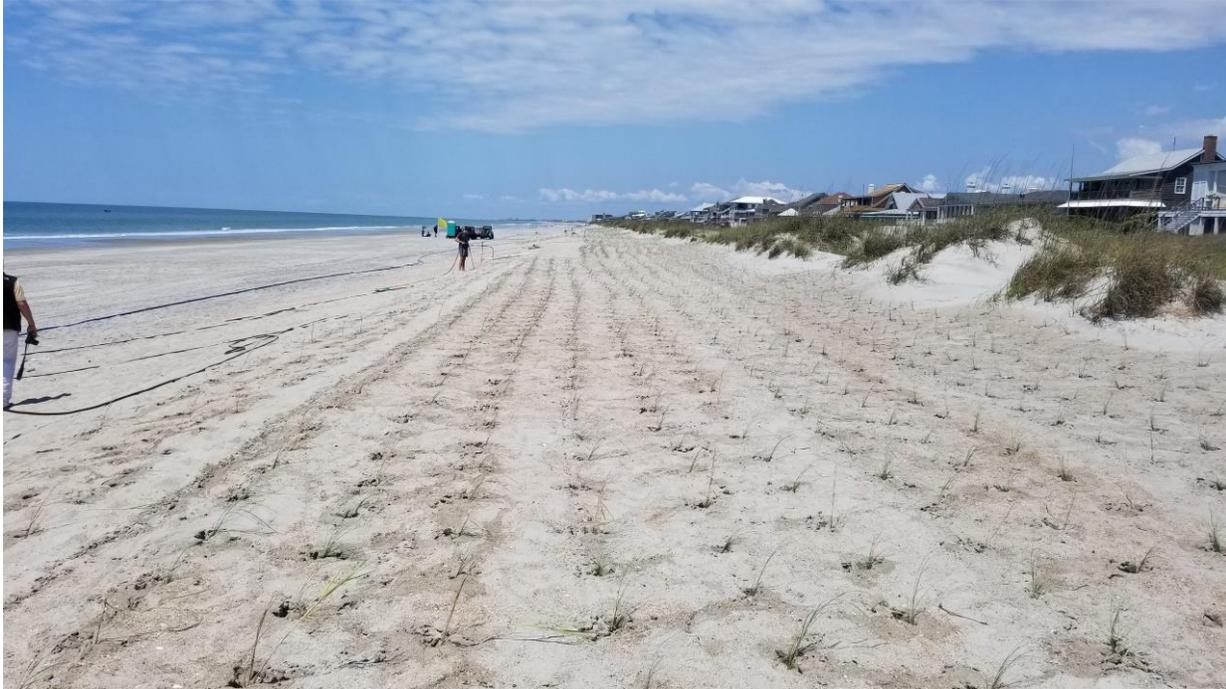
**Figure 2** – May 14, 2020, Atlantic Beach. The top (dune crest) of the newly constructed dune is planted with the aid of a mechanical planter, while the slope of the dune is planted by hand.
